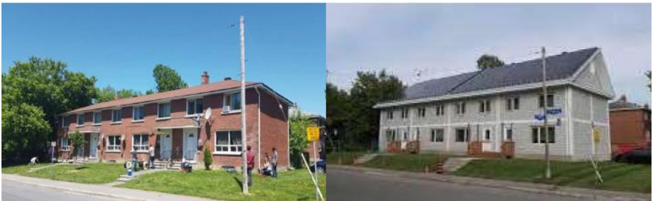
The Prefabricated Exterior Energy Retrofit (PEER) Pilot Project, Presland Road, Overbrook Community
